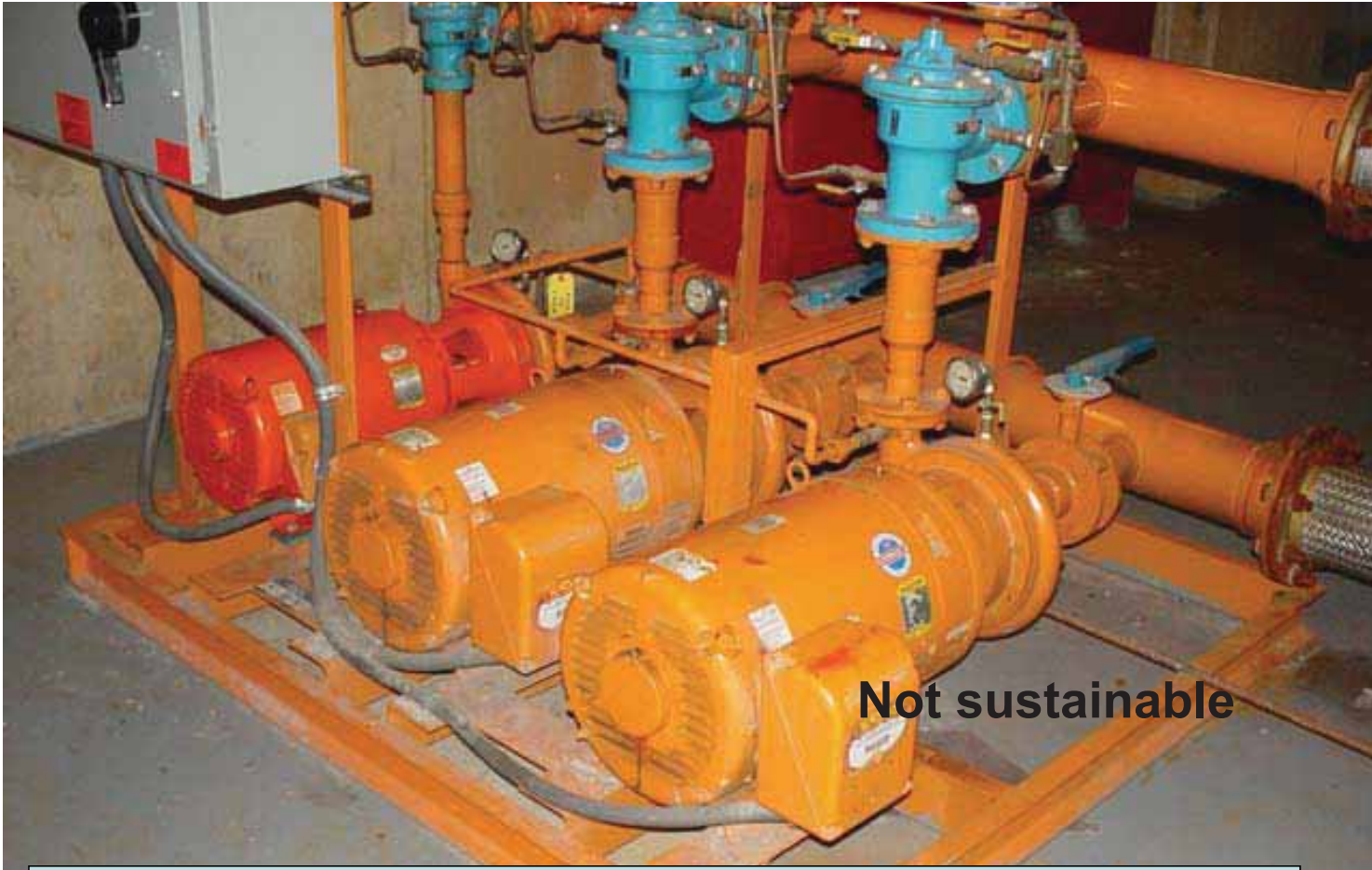
HW Recirc/Booser Pump Package # 2 of 3. Pumps & PRVs were replaced every 6 months
